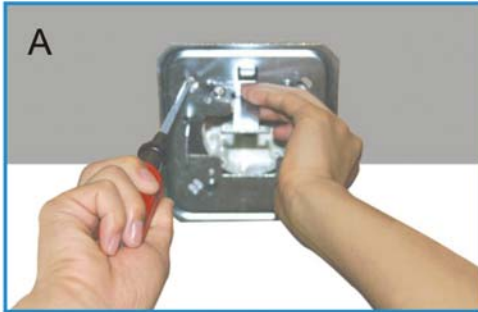
Mounting plate secured to standard J-Box
